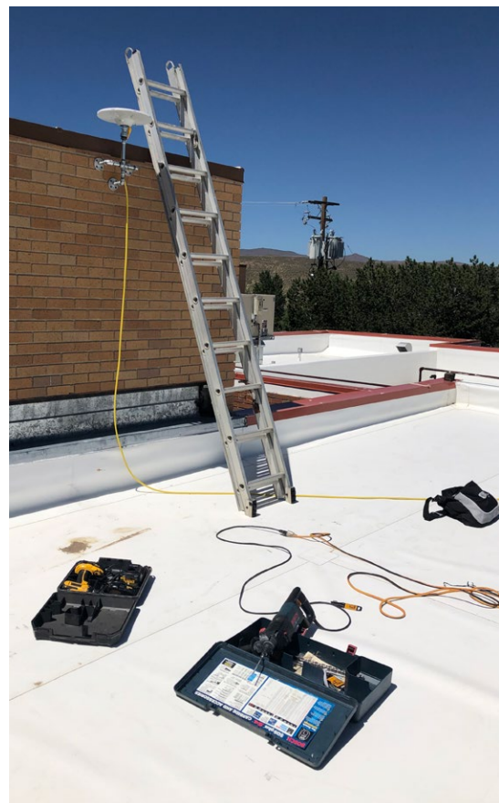
The installation site of a GNSS base station for The Utah Reference Network (TURN).
