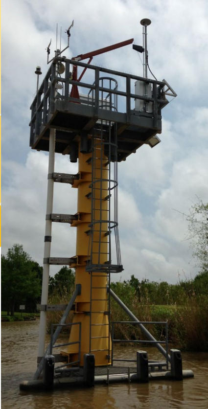
Located at Amerada Pass, La., this NOAA storm hardened tide gauge contains one of LSU C4G's GNSS base stations.
