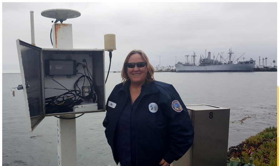
Kimberley A. Holtz stands next to a GNSS base station that withstands the harsh marine environment year-over-year at the Port of Long Beach, Calif.
